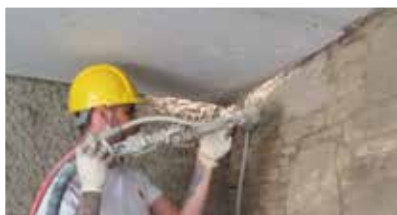
Installing internal wall insulation at retrofit project (Credit: Green Building Store)
