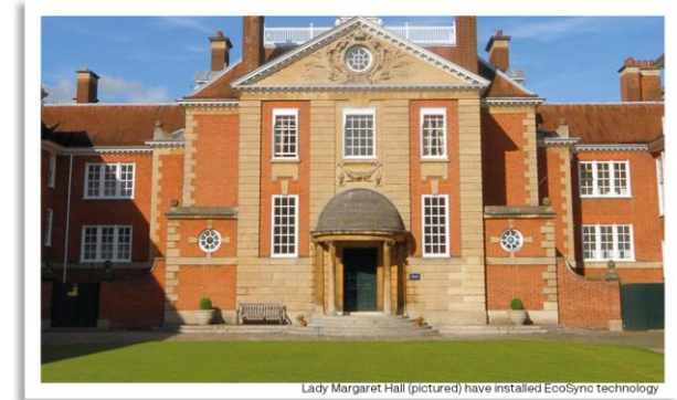
Lady Margaret Hall (pictured) have installed EcoSync technology
