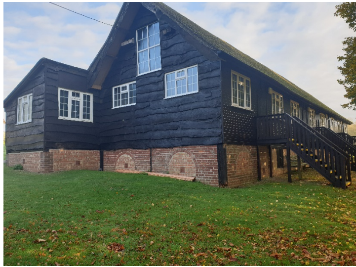
The new double glazing on one of Hill End's dormitories.
