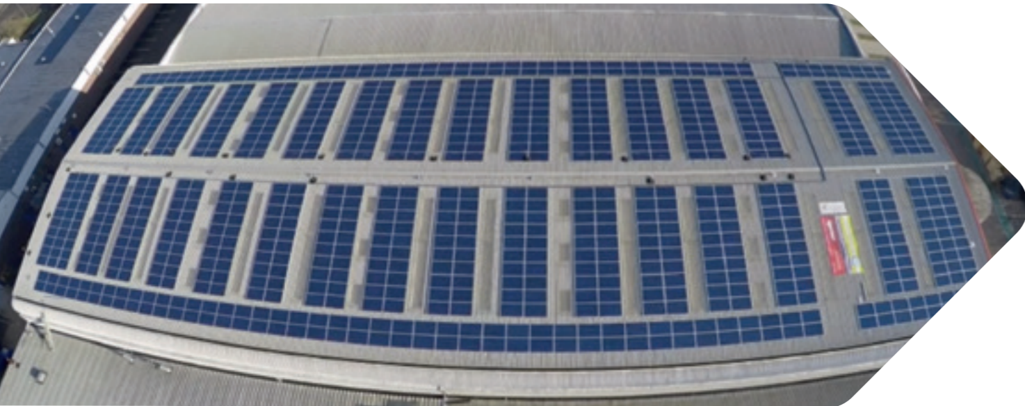
Solar roof at Norbar Torque Tools, Banbury (Credit: Low Carbon Hub)
