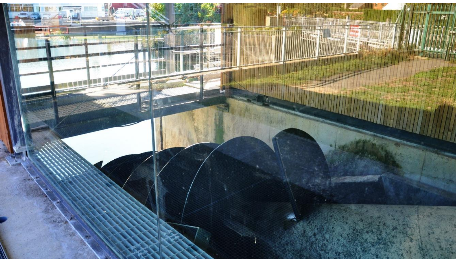
The Osney Mead Hydro project was supported with investment from the Greenfund
